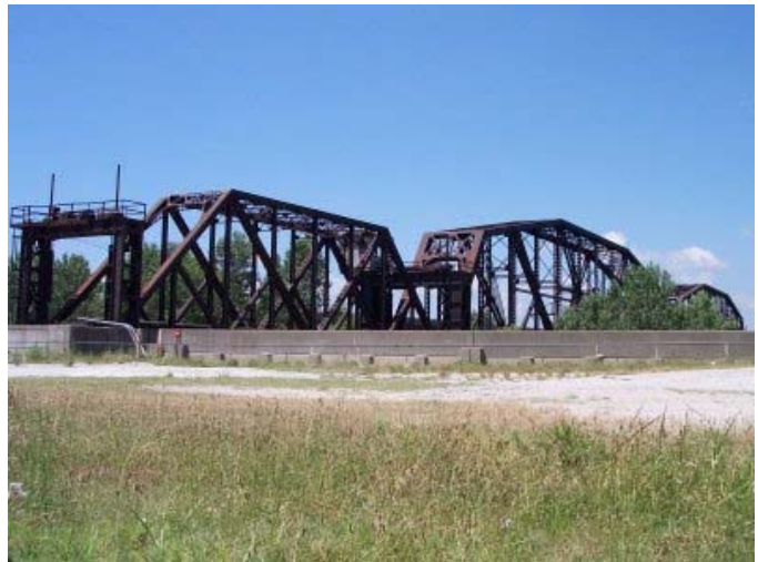
Γέφυρα Armourdale Rock Island
