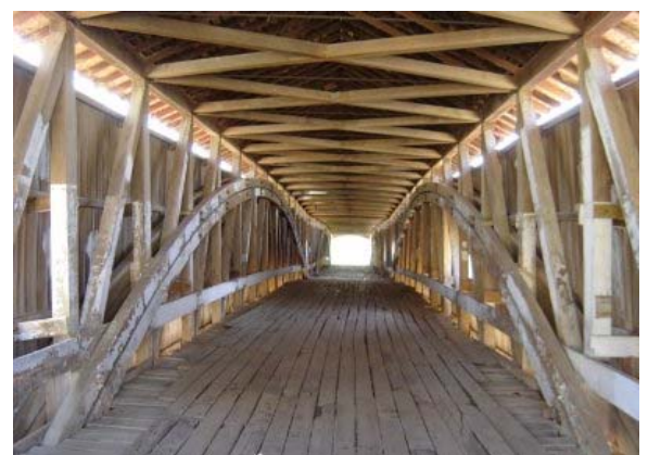
Γέφυρα West Union
