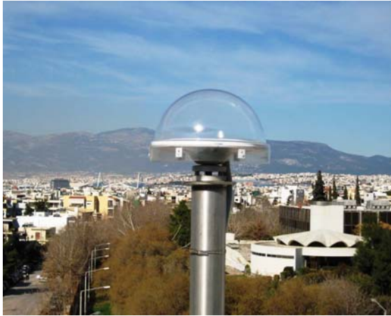
Fig. 3 A typical reference station of HEPOS.
