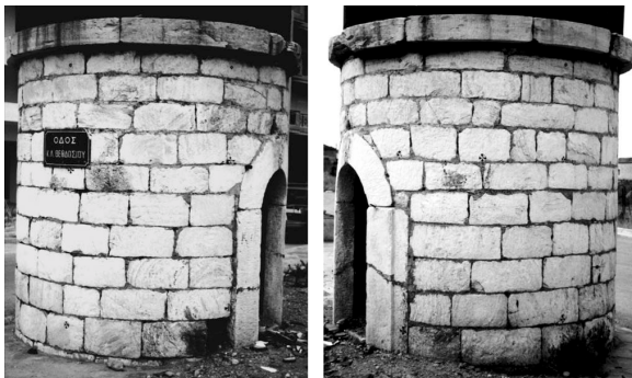
Figure 4 Two images of the water-tower.
