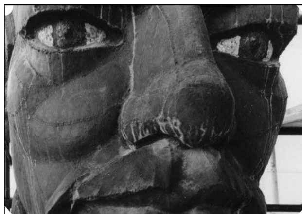
Fig. 5: Dark crusts on areas protected from rainfall.
