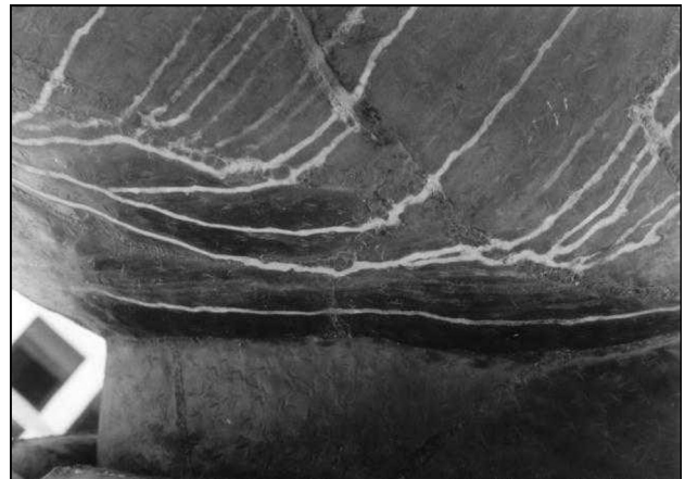
fig. 6: "Streaking" on the surface of the monument.
