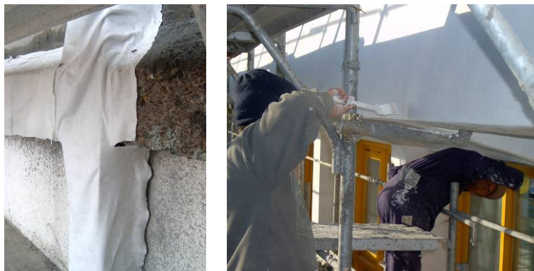
Figure 13-14. Protection of repair mortar by wet sheets and finishing by elastoplastic superficial protection.
