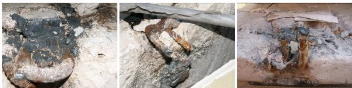
Figure 5. Corrosion of the hooks of lifting and connection of the infill panels and on the hooking systems of the same floors panels
