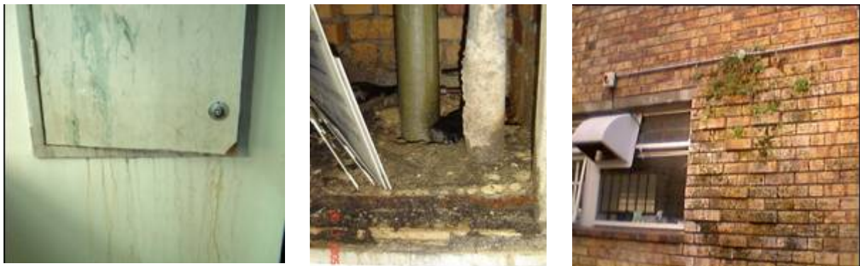
Figure 3: Duct to Service Duct, Inside Service Duct and External Wall outside Service Duct
