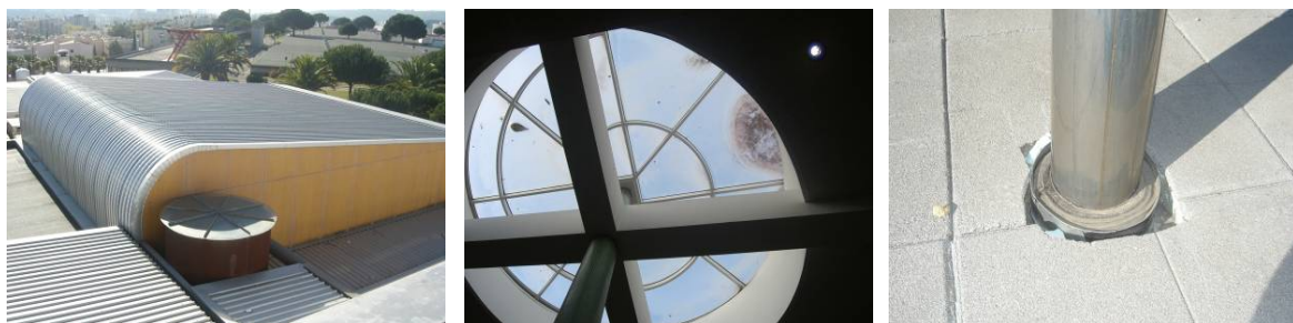
Figure 4. AF school - view of the gymnasium roof and the roof of the curling staircase which gives access to the upper observation gallery of the gymn where infiltrations were noted (left); VG school - infiltrations in the skylight (center); SB school - bad execution of the coating of the roof (right)
