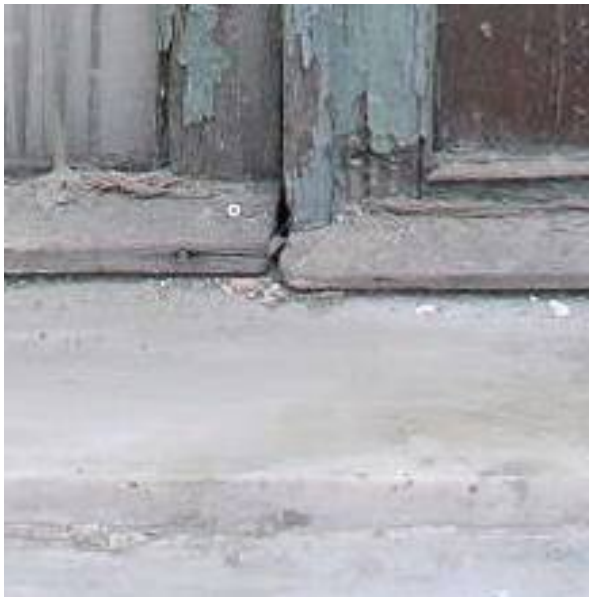
Figure 5. (a) Failure about the design of the connection point of doors and ground (b) Failure about the plumb line of the door
