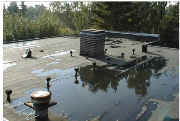
Figure 2. Example of a dead low-sloped roof with ponding water. Ponding water leads to a risk of reduced service life due to increased exposure of the roof membrane to moisture and freeze-thaw cycles.
