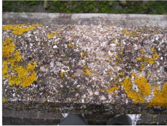
Figure 2. Typical condition and surface roughness of 1943 (left) concrete railing beams.
