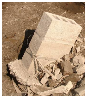
Figure 2. Foundation pier without evidence of mechanical connection.
