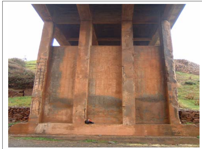
Figure 3. State of degradation of the bridge piles
