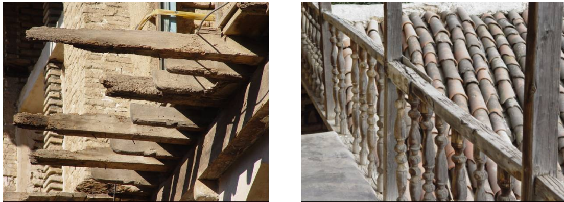
Figure 4. (a) Intensive weathering and (b) surface weathering, existing in House of Bagheri.
