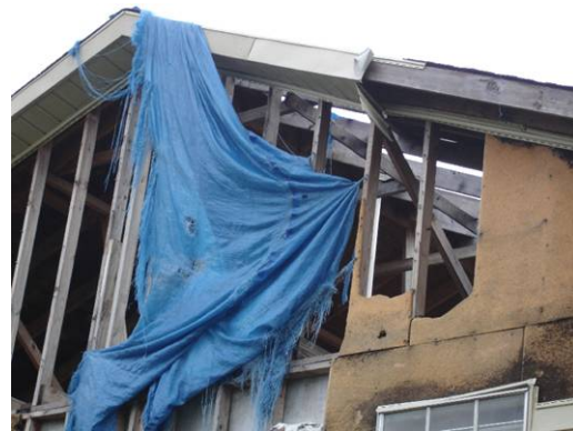
Figure 10. Poorly fastened sheathing that was blown off of a gabled end wall.
