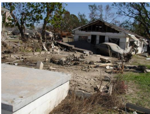
Figure 1. One story timber frame structure pushed away from the concrete porch.
