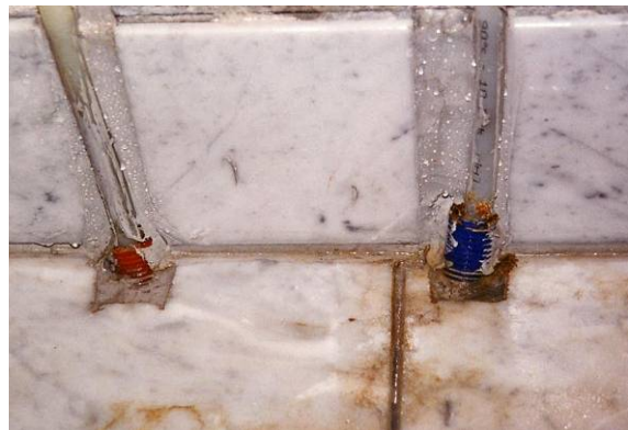
Figure 2. Example of pipe penetrations in a floor construction. The tubes (for the pipe in tube system) are finished just over the floor allowing water to run into the construction.
