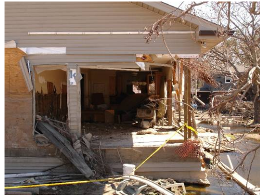
Figure 5. Wall clad with vinyl siding damaged in vicinity of a levee breach.
