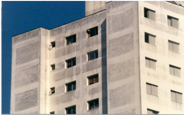
Figure 1. Dark stains caused by biological growth
