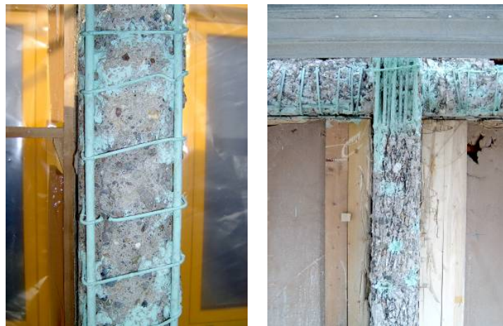
Figure 10. Application of the protect treatment of the steel bars against the corrosion.
