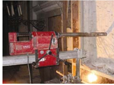
Figure 3. The HIUTI DD-250E coring machine dry
