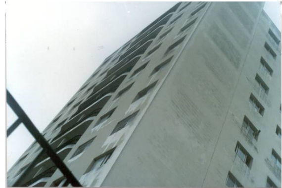
Figure 2. Areas with dark stains caused by rainwater, on the façade of the building
