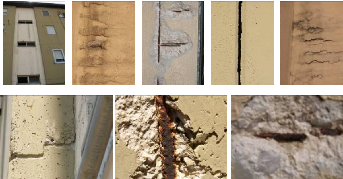
Figure 6. Expulsion of the layer protecting the steel road on the façade panels. Swelling and cracking of the plastic plaster
