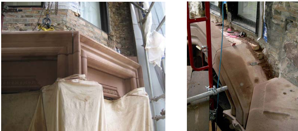
Figure 3. Representative example of new sandstone installation.
