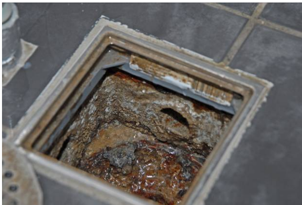
Figure 5. Example of new floor covering on top of the old. The floor gully has been extended with a plastic frame but unfortunately it is not watertight, see figure 6.
