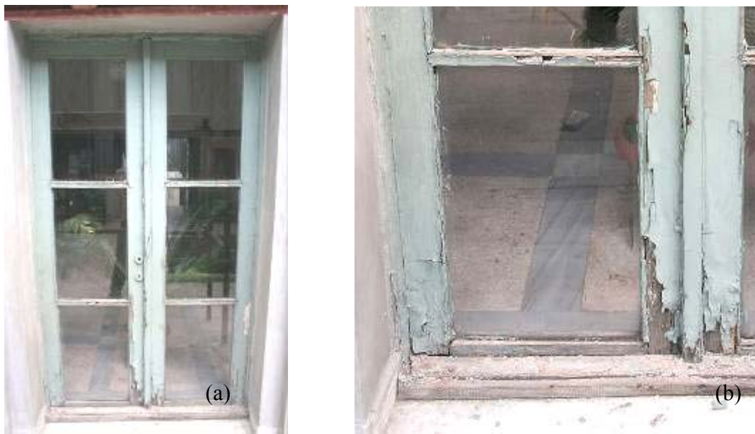
Figure 1. (a) The damage of the paints of the doors increases near to ground level (b) All of the horizontal elements of the doors are damaged
