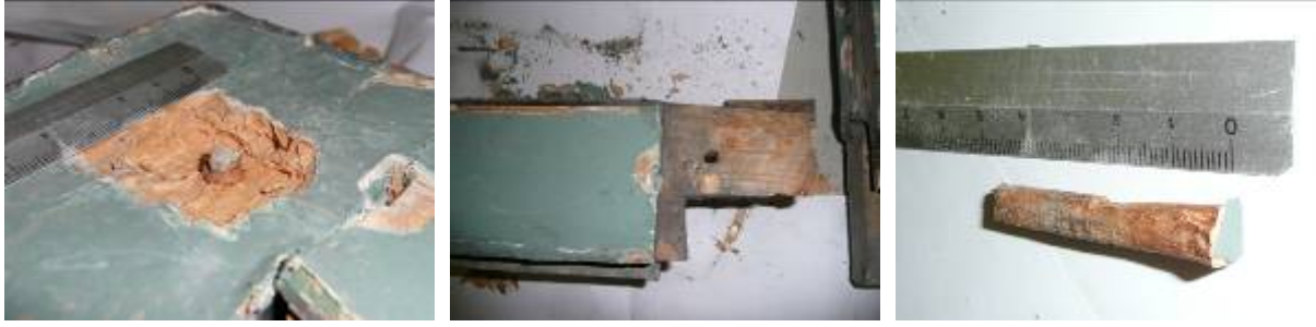
Figure 6. Detail of wooden nail for connection of the stud
