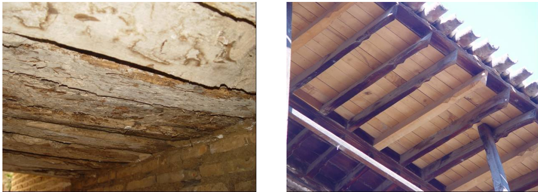
Figure 5. (a) Intensive decay and (b) new substituted rafters.
