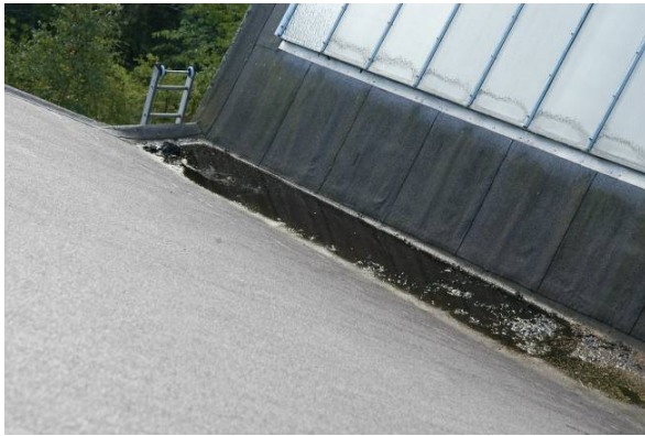
Figure 5. Example of ponding water in a valley. In this case the water remained in the valley almost permanently and, as a consequence, the protective granules were gone.
