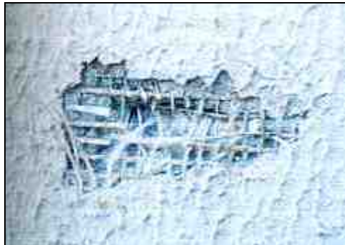
Figure 7. Vandalic damages, made easier for the lack further of specific reinforcing.
