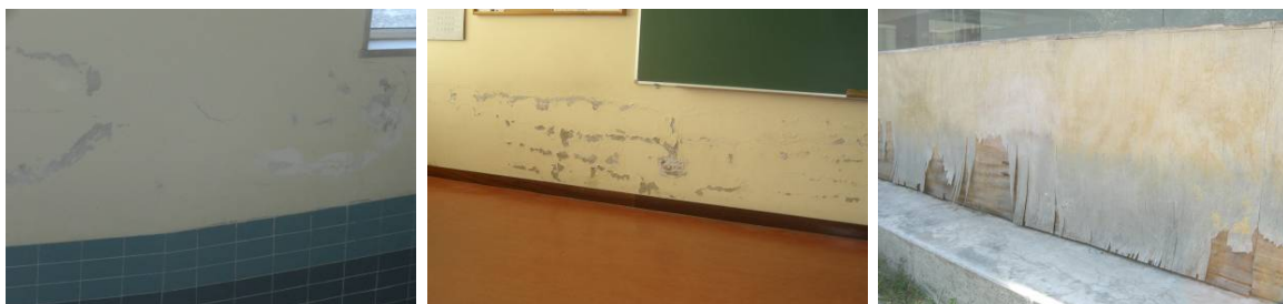
Figure 5. SB school: degradation of the interior coating of the bearing wall and the lower area of the classroom wall (left, center); AF school : very serious degradation of the exterior panel (right)
