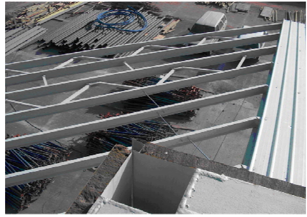
Figure 4. Mineral wool filling wall panels
