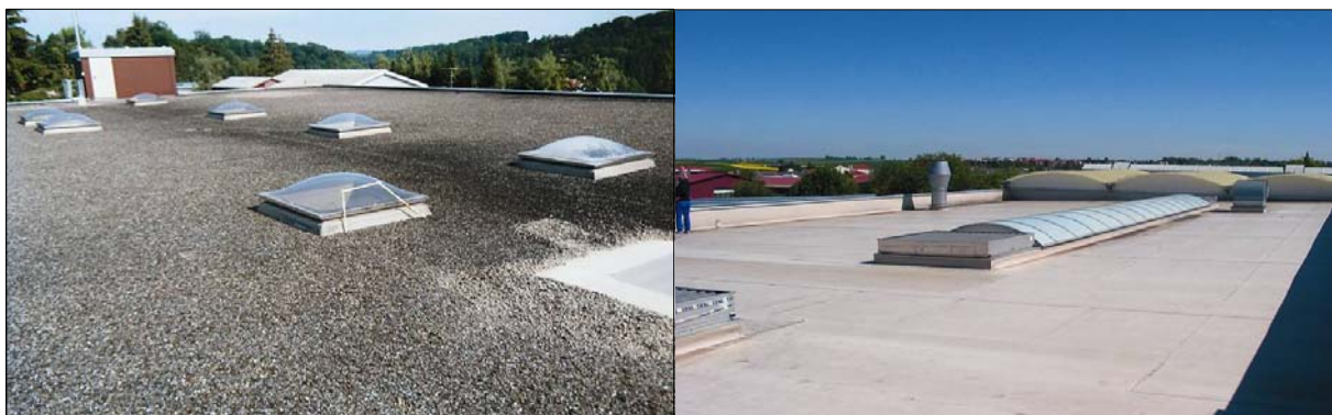
Figure 2. Two roofs investigated by Rieche [2004]. Left: Gravel ballasted industrial roof at Flawil, Switzerland (a typical application of G-type membranes). Right: Mechanically attached industrial roof at Ehingen, Germany (a typical application of S-type membranes).
