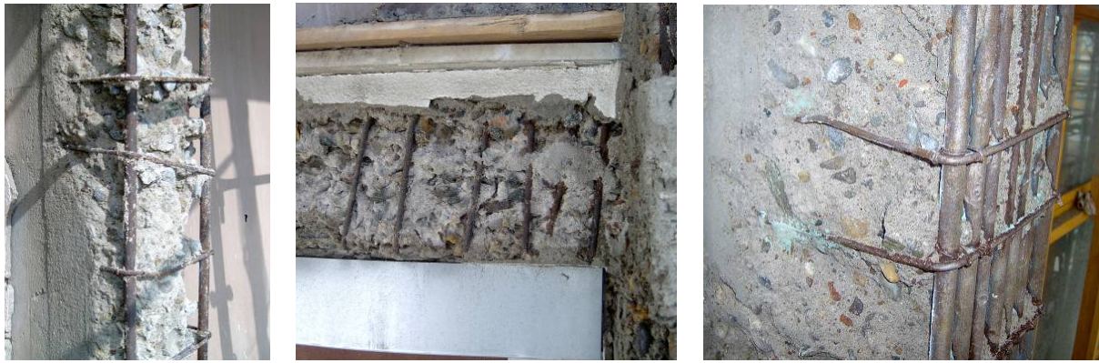
Figure 7-8-9. Comparison of steel bars cleaning: by mechanical demolition, by high-pressure water jets, by abrasive blasting.
