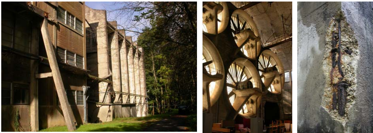
Figures 1, 2 and 3 : The air purifier (on the left) is an extension of the Meudon wind tunnel (in the center). It is locally very decayed, with large spalling areas (on the right) often linked to honeycombing.
