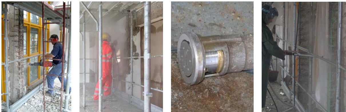
Figure 3-4-5-6. Removal of decayed material and roughening of concrete substrate by mechanical demolition and by high-pressure water jets.
