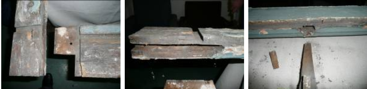
Figure 7. Detail of wooden connector for connection of the stud
