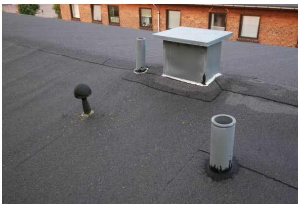
Figure 3. Example on different penetrating details normally seen on a roof.
