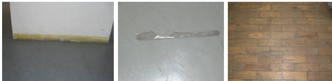
Figure 6. School 34 - absence of a baseboard due to loss of adherence (left); AF school - detail of the wear and tear of the central atrium's floor covering (center); VA school - deficient maintenance of the floors of the rooms (right)
