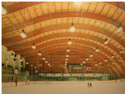
Figure 4. Glulam and plywood roof system of Disney Ice, in California, create a modern sculptural quality and recall traditional [APA, 2002].
