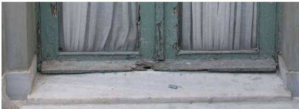
Figure 2. Decay in the components near to ground level.
