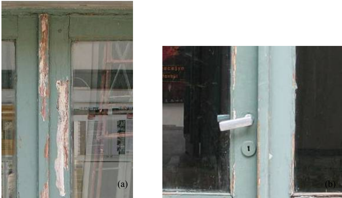
Figure 3. (a) Damage on the surface of wooden components of doors. (b) Deformation of door handle.
