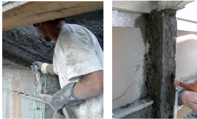
Figure 11-12. Application of the mortar mechanically sprayed (by wet-mix shotcrete) and finishing by hand with plastering trowel.
