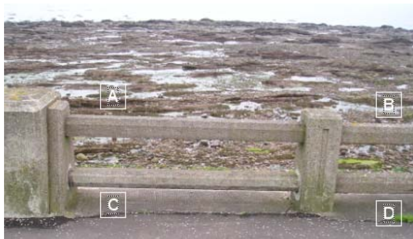
Figure 1. Typical (part-)section of the RC promenade railing showing the four precast railing beams, the cast-in-situ central support and the left end-post.
