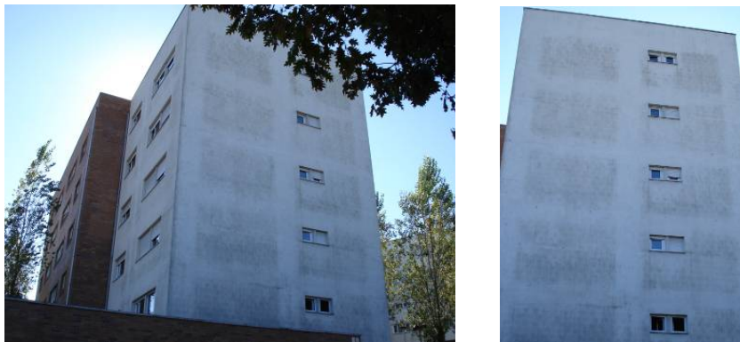
Figure 1. Building covered with ETICS showing microbiological growth.
