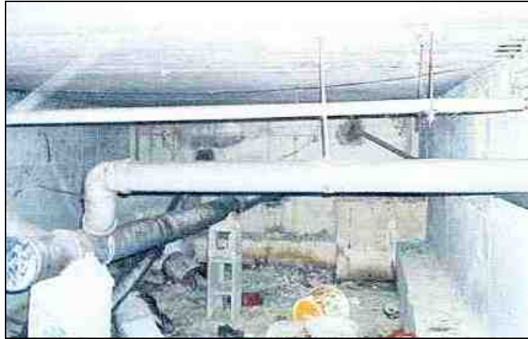
Figure 6. Hollow space under first floor, with signs of flood and great humidity ratio. On the top, right-hand, steel bars spelling concrete cover.
