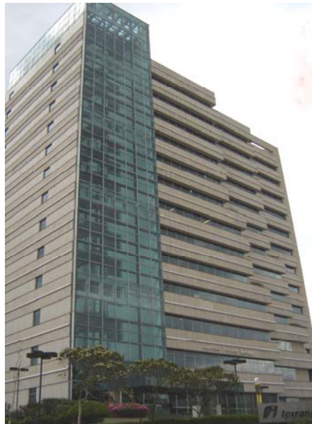
Figure 5. Transparent facade displaced from the structure.
