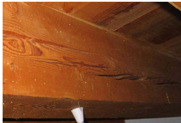
Figure 9. Drying cracks in timber beam affecting shear capacity
