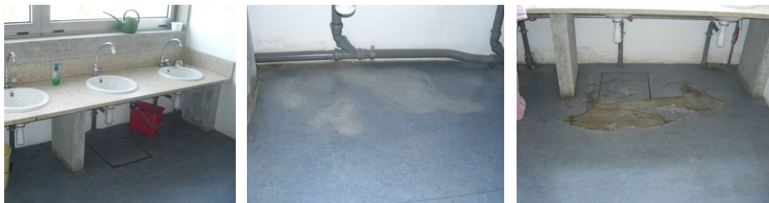
Figure 8. School 34 - effect of the permanent water leaks on the floor covering
