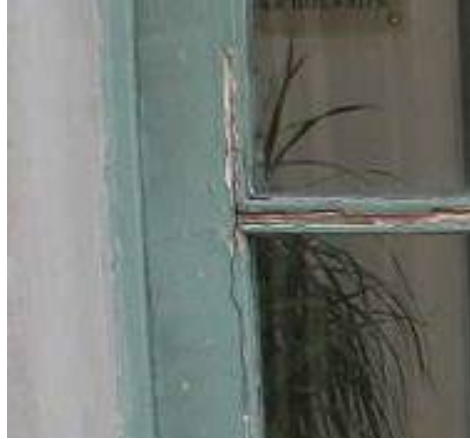
Figure 4. Failure about the design of the connection point of glass and wooden components of door
