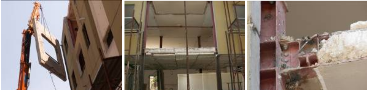
Figure 2. Bearing structures of buildings and non carrying infill prefabricated panels of façades
