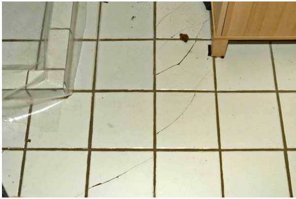
Figure 3. Example of cracks in a floor with underlay of plywood but with insufficient stiffness.
