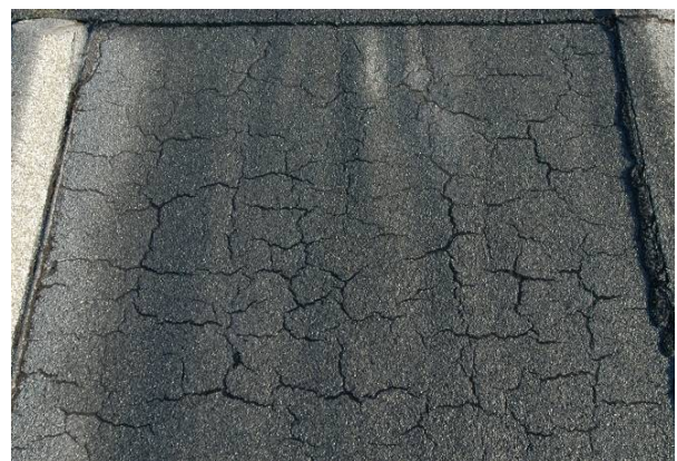
Figure 4. Superficial "cracking" in the bitumen on steep surfaces leads to reduced protection by the granules.
