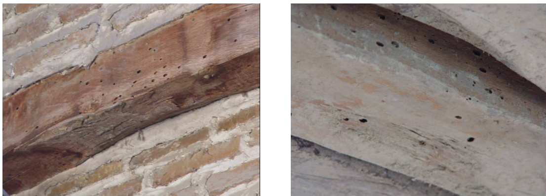
Figure 7. Holes due to insects attack
