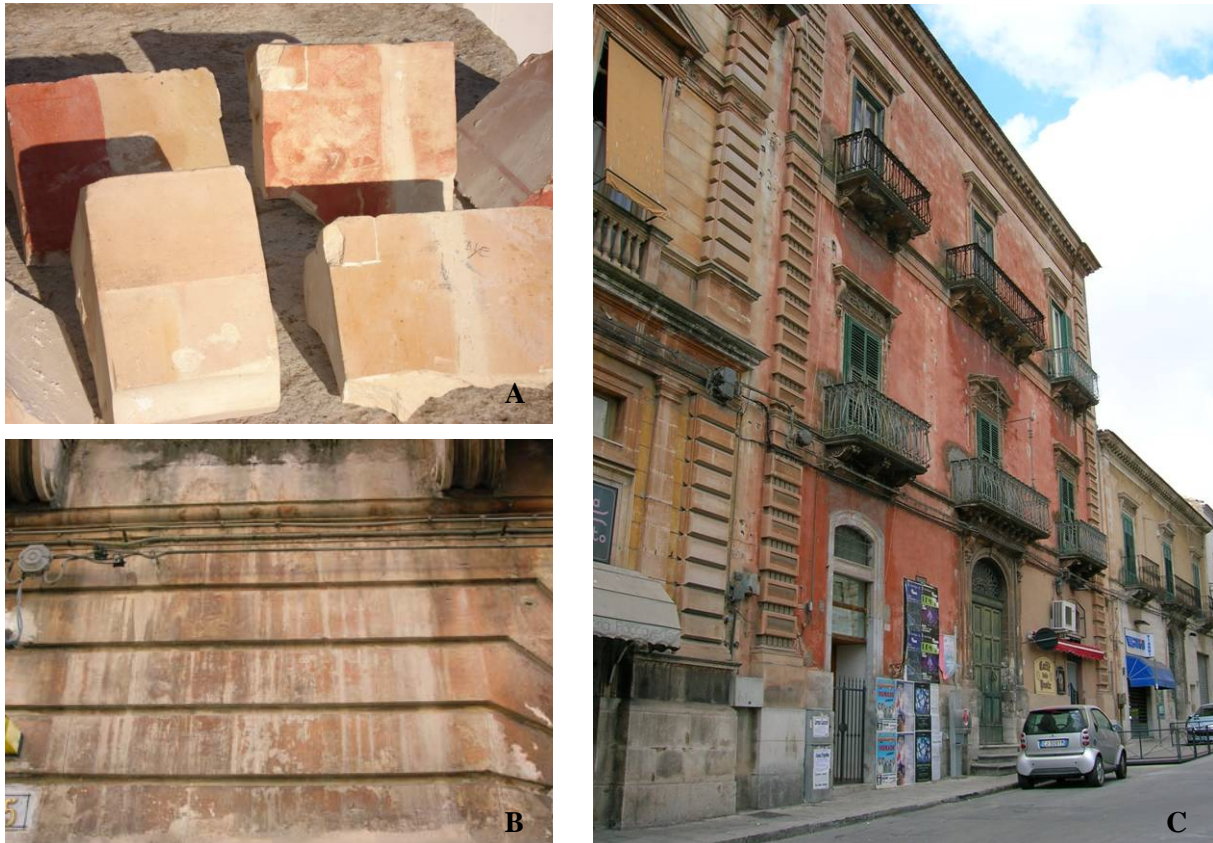
Figure 3. A: Samples of light coverings with linseed oil and natural earths.; B: Plastering with lime water and natural earths.; C: “Lime paint” on plaster (lime milk and oxides).
