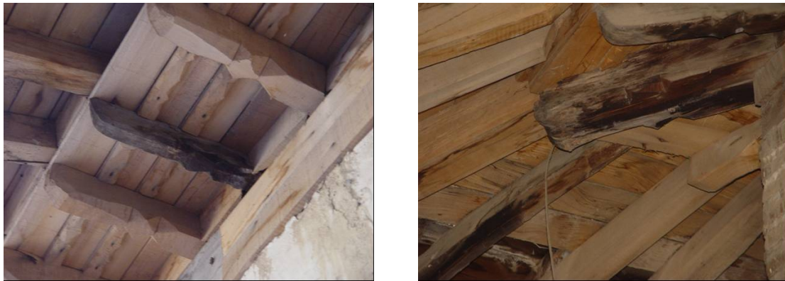
Figure 6. Existing moisture-related problem in new member
