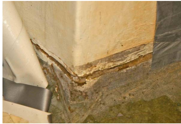
Figure 4. Example of insufficient welding – worst example ever seen – with repair of the joint with tape. Probably a do-it-yourself work.
