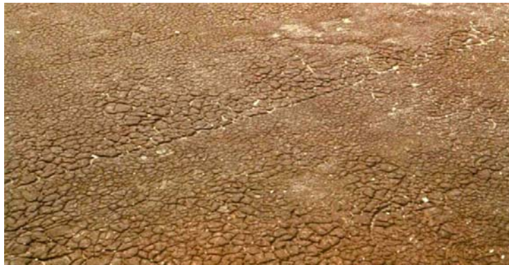
Figure 5. Example of unprotected bituminous waterproof membrane (courtesy Prof. Alexandru Stan).
