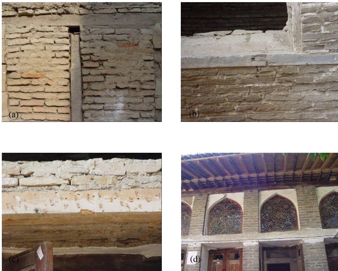
Figure 3. The main construction materials used in House of Bagheri, (a) brick and cob, (b) solid wood beneath the door, (c) solid wood up the door and (d) solid wood as main beam and rafters.
