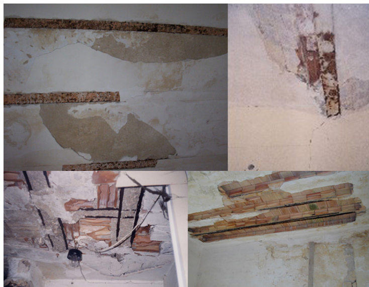
Figure 2. B2 type floor: plaster detachment and impost brick breaking; C1 type floor: concrete elements detachment and bricks breaking.
