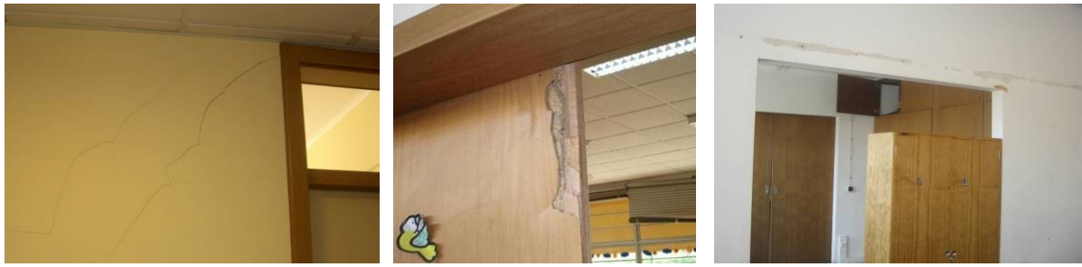
Figure 7. SB school - detail of the cracking of the walls of the ground floor (left); VA school - detail of a door deterioration (center); school 34 - removed sliding doors (right)
