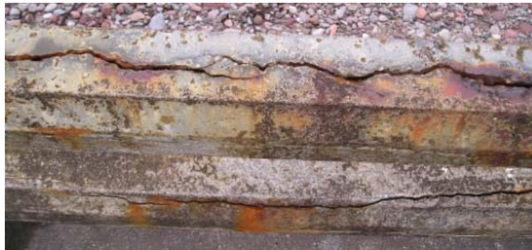
Figure 3. Typical crack pattern in 1993 railing beams
