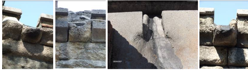
Figure 10. The spouts, WS1, WS4, WS5 and WS7 (from left to right, respectively) showing the severely-deteriorated sluiceways due to cement-based mortar repairs [Disli et al. June 2007].
