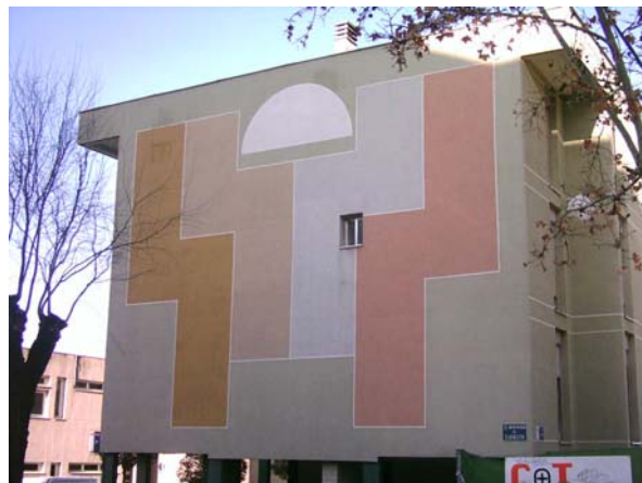
Figure 7. ETICS with XPS after ~15 years of service. No cracks nor blisters are detectable. (Photo: residential buildings in Guadalajara/Spain ).
