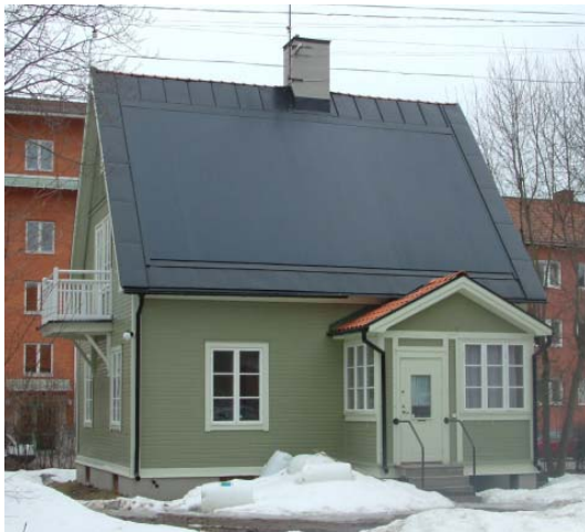
Figure 1. The Swedish demonstration site (Endosite) in Sandviken, showing the roof integrated USC. A drawing showing a top and bottom isometric view of the roof integrated USC used in the Swedish demonstration site (Sandviken).
