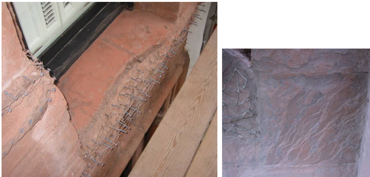
Figure 1. Representative example of previous repair which has subsequently failed and face bed unit.
