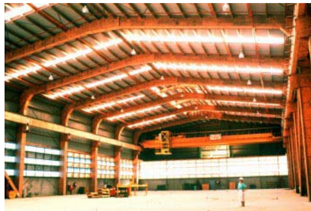
Figure 8. The use of LVL at the store building in Australia [Ferguson, 2006].
