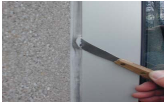
Figure 3. This is an example of the type of “invisible” seal failure uncovered by using the non-destructive method and device described elsewhere in the paper. Prior to finding this seal breach, the entire sealant bead depicted looked exactly like the area above and below the breach.
