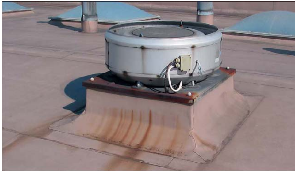
Figure 3. Curb flashing detail, industrial building at Ehingen, Germany.
