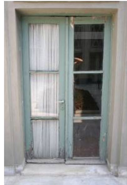
Figure 5. (a) Failure about the design of the connection point of doors and ground (b) Failure about the plumb line of the door
