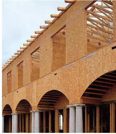
Figure 9. Use of OSB in wall sheathing, roof sheathing, and floor sheathing [LP Building Products 2005].
