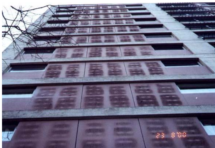
Figure 1. Building facade with microorganism development
