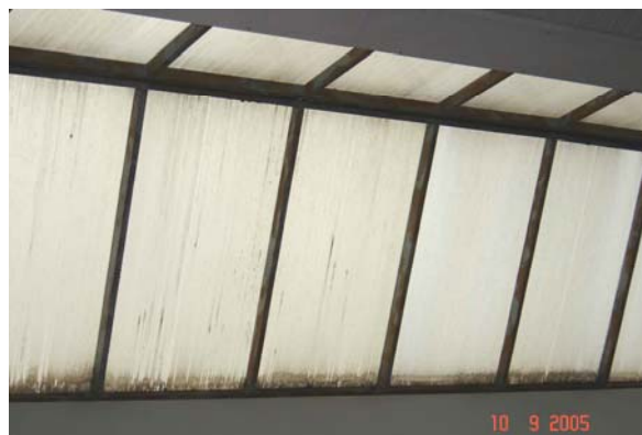
Figure 4. Glazing with alveolar polycarbonate with build up of dust.
