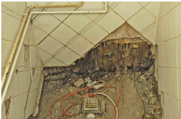
Figure 1. Example of a bathroom wall made from wood based material without a watertight membrane. The lack of watertightness resulted in a total renovation of the bathroom due to fungus and dry-rot in the constructions.
