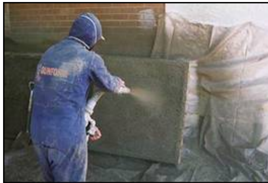
Figure 2. Spraying distance and angle were kept around one meter and 90°, respectively.
